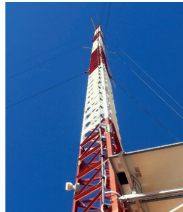
DTBird® Detection Module installed in a meteorological tower. 2 to 8 HD Cameras can be installed per tower.
