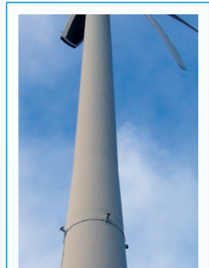
DTBird® Collision Avoidance Module Speakers installed on the WTG tower. 4 to 10 Speakers can be installed per WTG.
