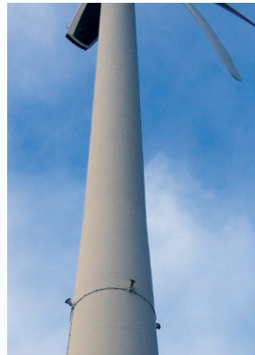
DTBird® Collision Avoidance Module Speakers installed on the WTG tower. 4 to 10 Speakers can be installed per WTG.
